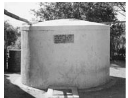
Hand constructed Water Cistern
